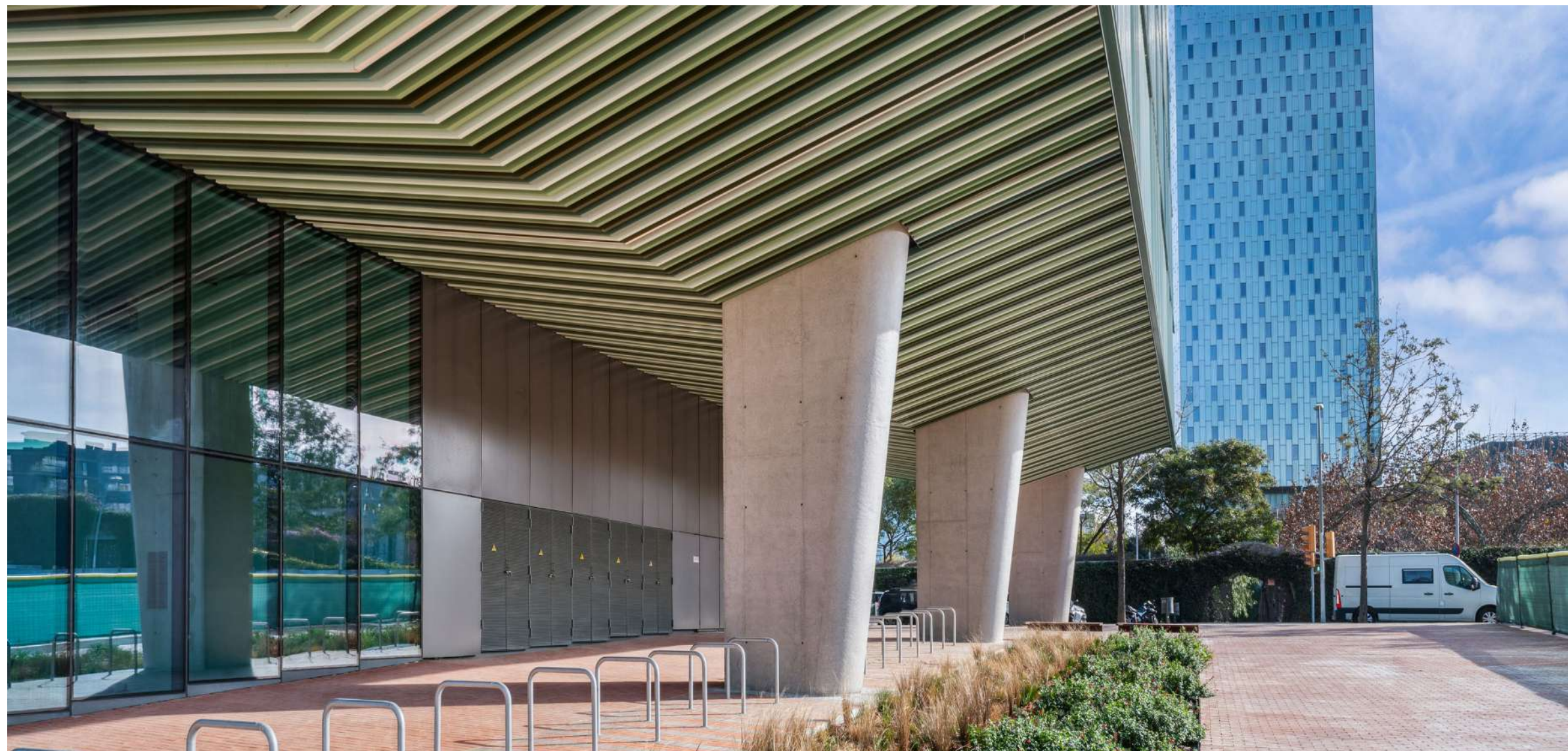
Lobby and bike parking
